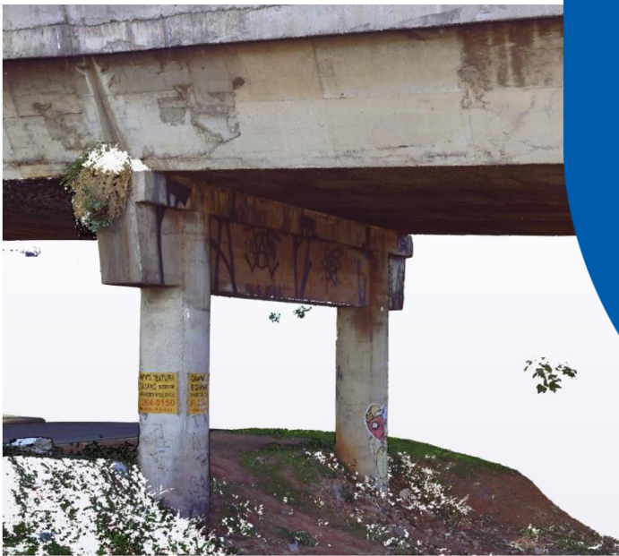
Laser Scanner Terrestre
