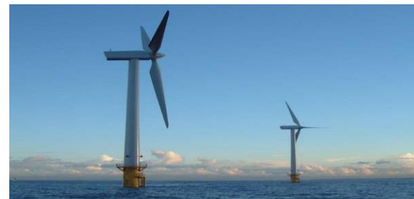
Offshore Wind Monopiles
