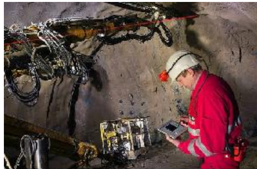
Setting out of drill holes by WLAN-Interface
