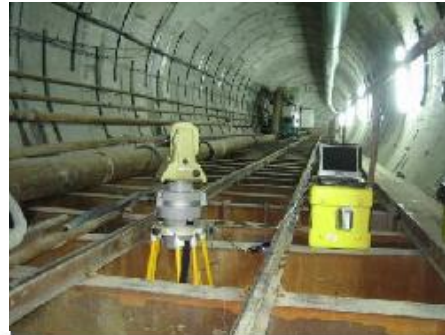
Gyro-measurement in a subway tunnel (Metro Sofia, Bulgaria)
