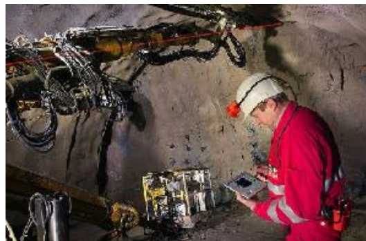
Setting out of drill holes by WLAN-Interface
