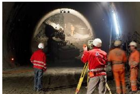
3D-displacement measurements with free stationing during excavation
