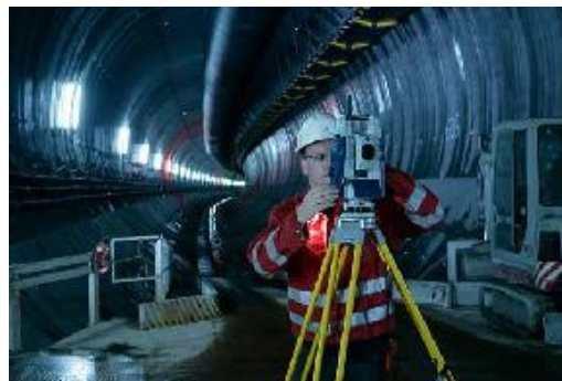
Control of the tunnel network for excavation (Tunnel Chain Perschling, Austria)
