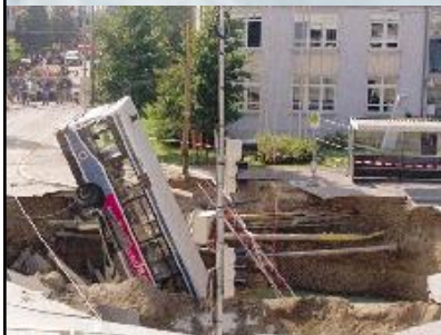
Chimney Failure, Munich
