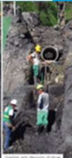
Installing and shaping of ditch
