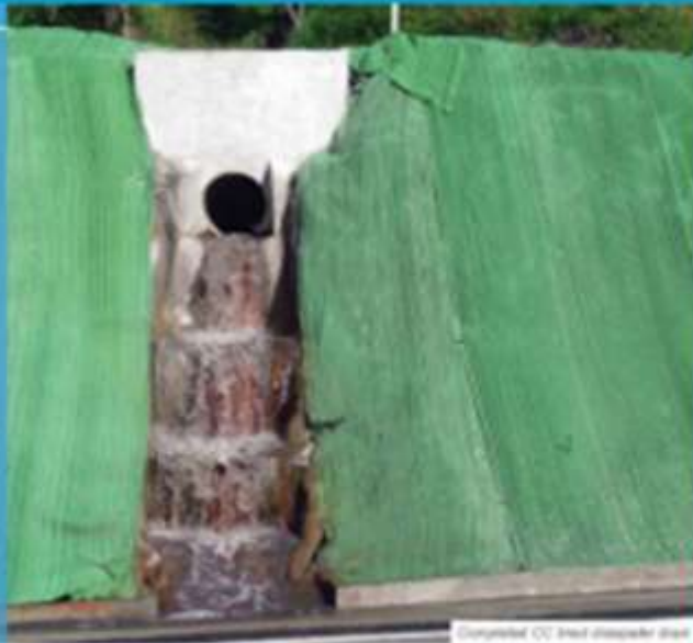
Completed CC ditch drainage ditch
