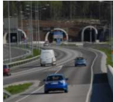
OBJECTS (BRIDGES, TUNNELS, LOCKS)
