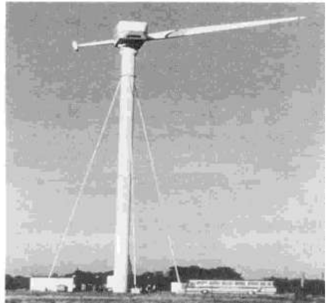
Figure 7.19 Single-bladed HAWT (MBB 600 kW turbine)
