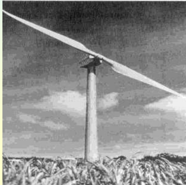
Figure 7.17 Two-bladed HAWT (WEG MS400 turbine)
