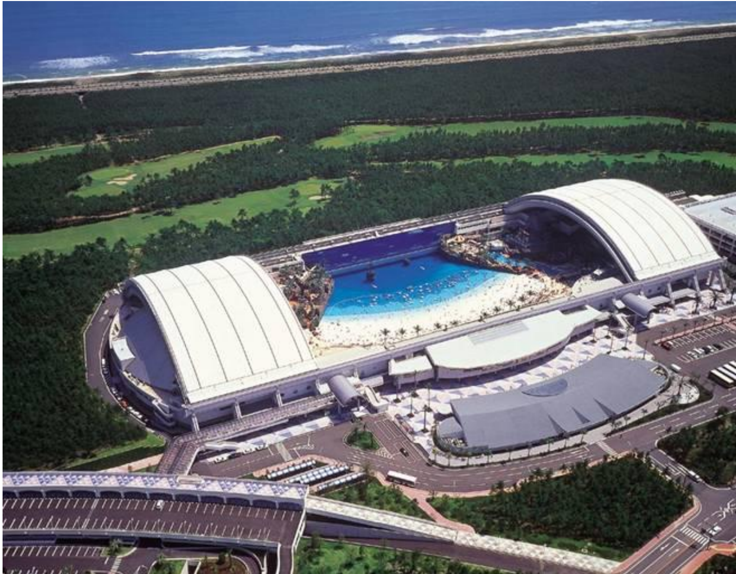
Ocean Dome, Japan the world's largest indoor water park (300m-100m-38m), with a retractable roof.
